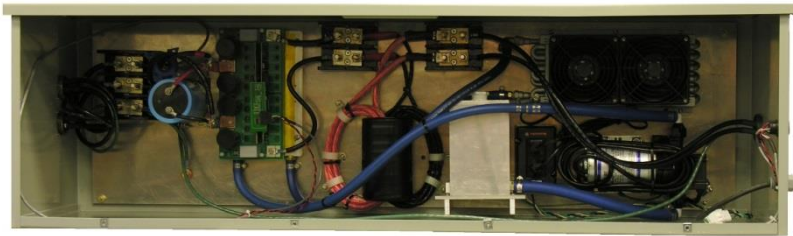
HF inverter system with HF transformer and self contained thermal management system
