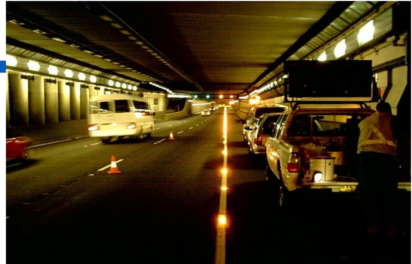
Tunnel (Sydney Australia)
